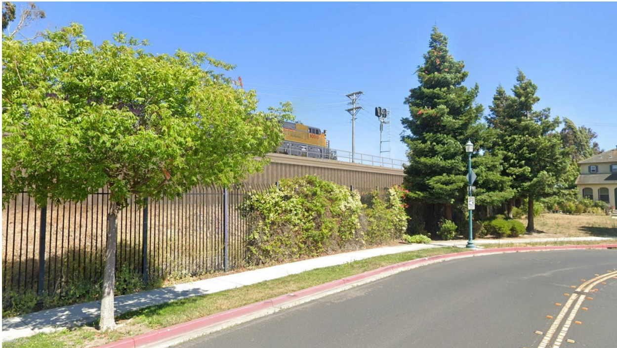
Figure 3.2-14. Viewpoint D – View of the Coast Subdivision tracks, looking east from Novato Street (Proposed Project)
